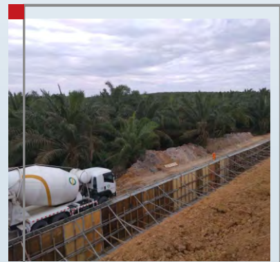
PENAHAN TANAH RETAINING WALL
